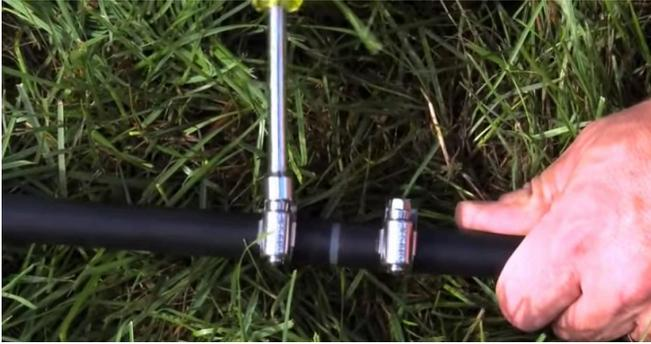
Unroll the EasySet™ weighted airline and remove any kinks or twists. Join enough sections of weighted airline, using 3/8" or 5/8" connector kits, so that the airline can rest on the bottom of the pond, from the pond's edge out to the planned location for each diffuser. For option B installations, connect the weighted airline to the direct burial airline or Remote Manifold Kit at the pond's edge.
