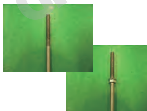
11. The nut on the battery j-bolt will be installed upside down so the brace is mounted properly.
