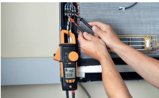
Measuring voltage on an air conditioning unit with testo 770 .
