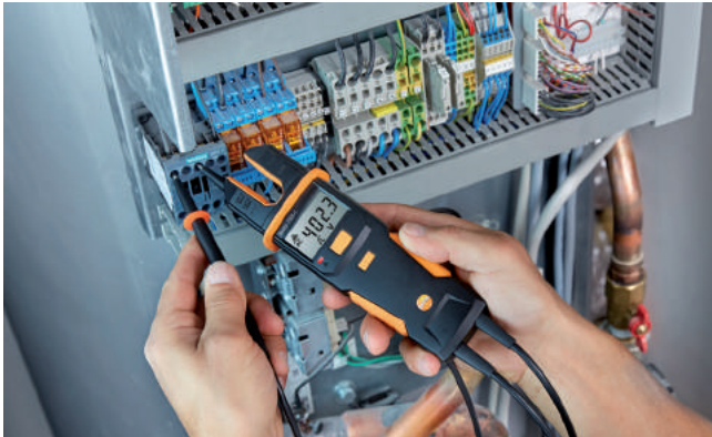
Testing voltage on a heat pump with testo 755 .
