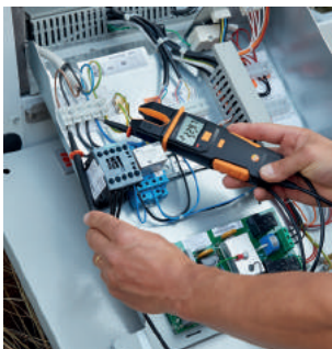
Measuring voltage on a compressor.
