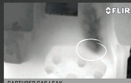
CAPTURED GAS LEAK
