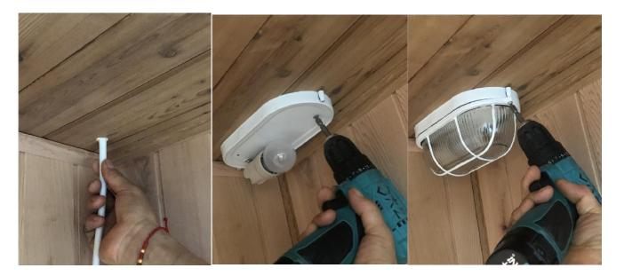
Attach the dome light to the back wall of the sauna in your
