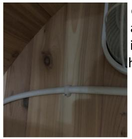
desired location. Run the white wire around the edge of the sauna using the included clips and attach it to the heater per the electrical instructions.
