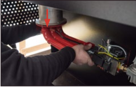
5 - Remove the burner from its housing
