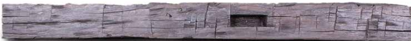
Hewn Mortise Beam
