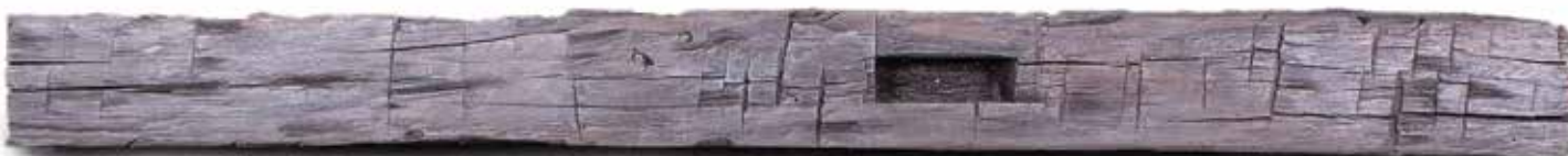
Hewn Mortise Beam
