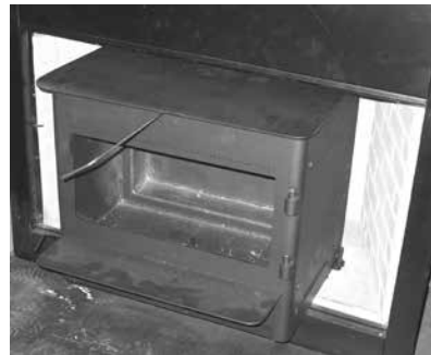
Pull Rod in place Diagram 6
