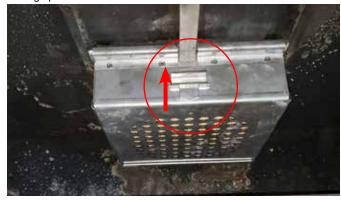
8. Pull flame shield forward and tilt down, be prepared to support catalyst assembly.
