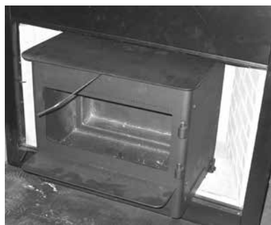
Pull Rod In Place
