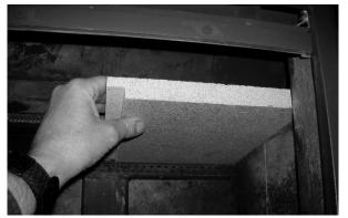
Figure 18 (cont.) - Removing/Replacing the Baffle for Inspection
