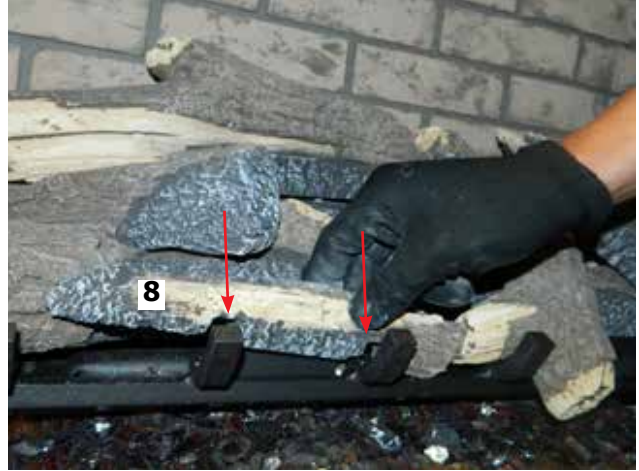
Diagram 14—Install Log 8
