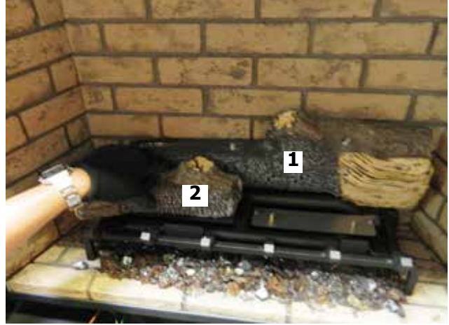
Diagram 8—Install Log 2
