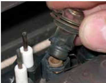
Diagram 2: Slide burner assembly to the right—then remove.
