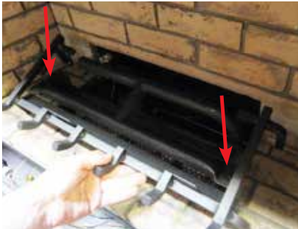
Diagram 1: Remove the left and right screws.
