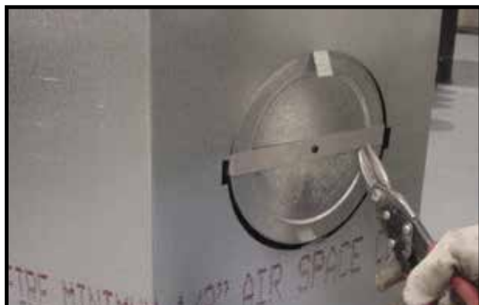
Figure 6.10 Cut the metal retaining band and fold the sides out.
