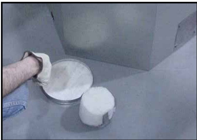
Figure 6.12 Discard the seal cap, remove and discard the insulation basket.
