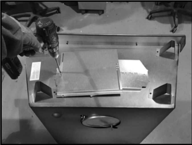
Figure 6.1 For top vent, remove the screw holding the elbow heat shield in place.
