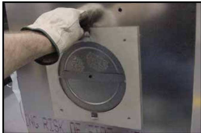
Figure 6.9 Fold the tabs toward the center of the fire plug (90°) and remove the insulation gasket.
