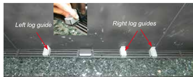
Log guides installed
