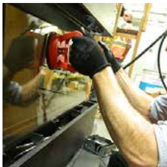
Handle glass with supplied vacuum clamps
