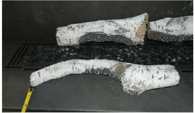
Log 4 —2" to end of front panel
