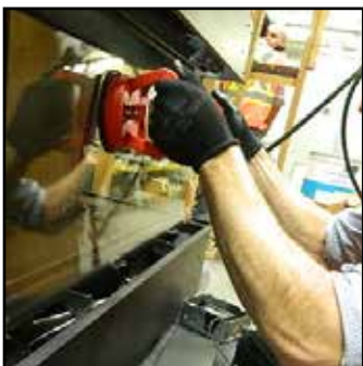
Handle glass with supplied vacuum clamps
