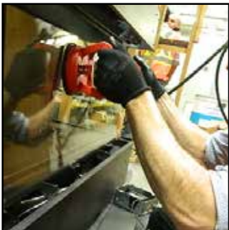
Handle glass with supplied vacuum clamps
