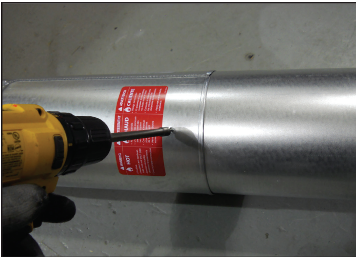
Figure 7.4 - Screws into Slip Section
