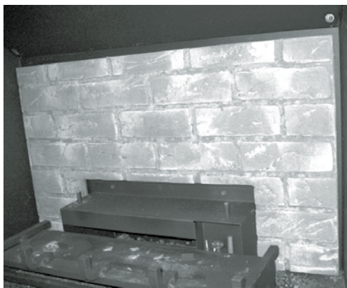
Back Panel Installed
