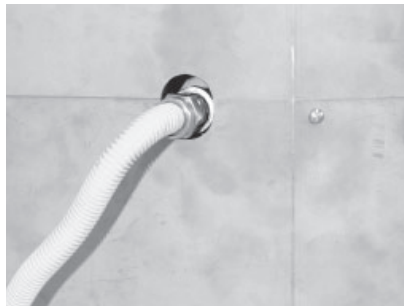
Flex connector redirected using one elbow.
