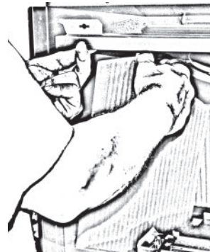
Rotate anchor up and insert panel
