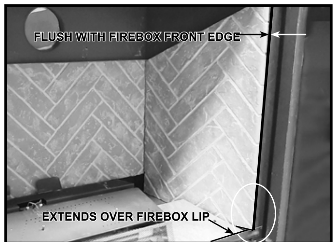
Figure 11.4 Side Refractory Panel Installed (Right Side Shown)
