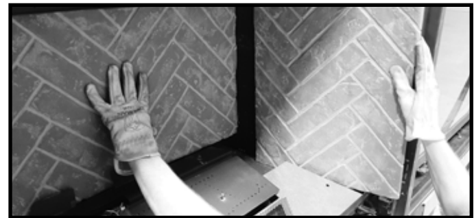
Figure 11.3 Install Side Refractory Panel (Right Side Shown)
