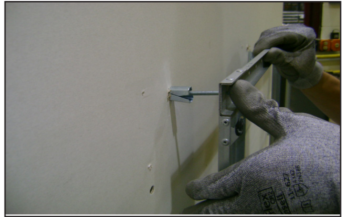
Figure 4.6 Installing Anchors in Hollow Wall
