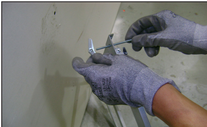
Figure 4.5 Toggle Bolt Installation through Mounting Bracket
