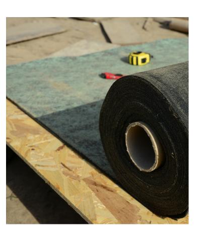
Ensure you pull the felt taught so that it is flat against the roof. When you get to the bottom edge, hammer the nails in at 30cm intervals.
