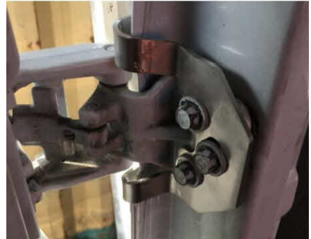
Figure 5: Inside View of Installed Upper Hinge
