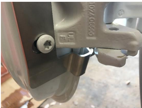
Figure 5: Installed Lower Hinge Bracket
