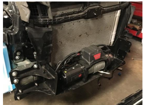
Figure 27: Winch Installed onto Winch Plate
