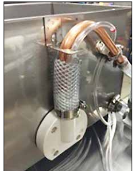
Air gap configuration prior to S/N G200325482.
