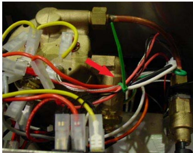
Figure 24. Tie up the cables.
