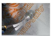
4. Fasten the insulation board on the wall mechanically with a couple of nail clip plugs (stone wall) or timber screws (timber frame wall). Mechanical fastening and the foam sealant ensure a strong adhesion of the insulation board to the wall.
