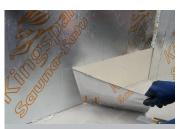
11. Remove the aluminum foil from the insulation surface on the area of the socle tiling. The aluminum foil is easiest to remove from the side where the board's code text is printed.
