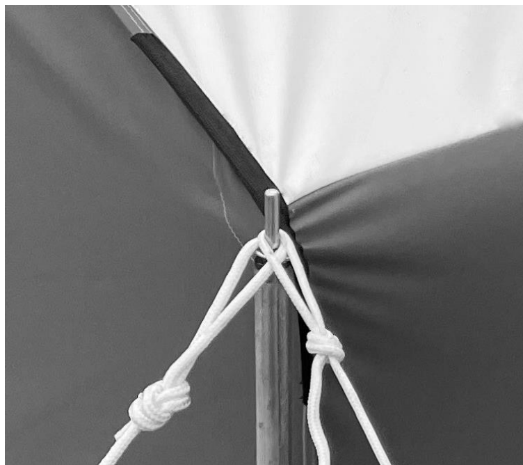
Fig 4. Side Upright Pole at Corner
