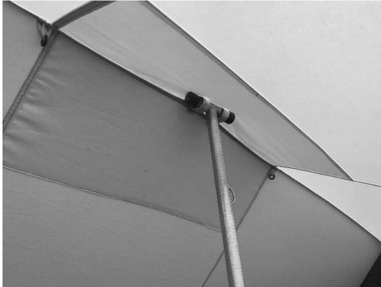
Fig. 7 Center Support Pole Installation
