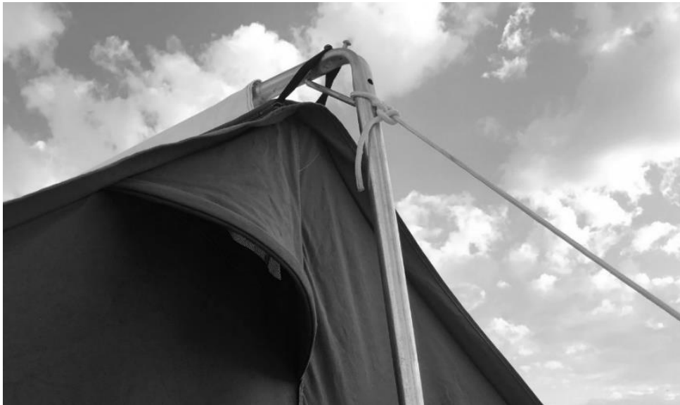
Fig. 2 Main Upright Pole Connecting to Ridge Pole
