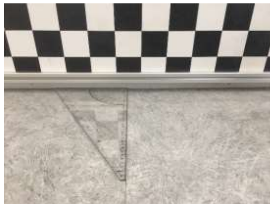
Finding a line perpendicular to the wall
