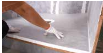
Embed the tray in the mortar
