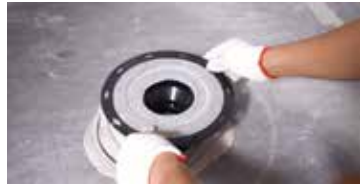
Press the bonding flange into the mortar
