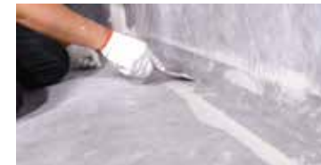
Make the surface even
