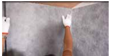
Finish covering the membrane
