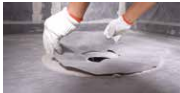
Cover the waterproofing membrane
