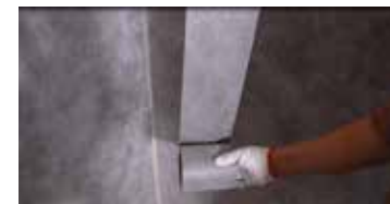
Prepare the waterproofing strip
