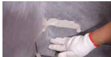
Install the waterproofing corners 1
