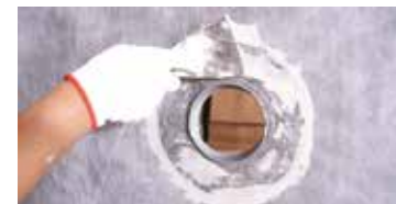
Trim the pipe seal
