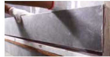
Fix the curb firmly
