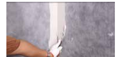
Brush the mortar on the corner
