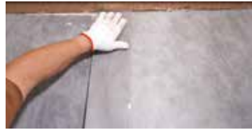
Cover the waterproofing strip on the joint
