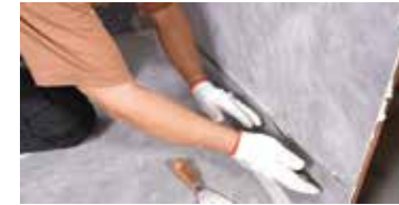
Cover the waterproofing strip
