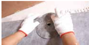
Cover the mixing valve seal
