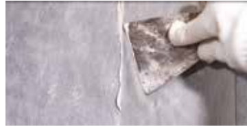
Make the wall surface even
