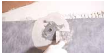
Make the surface even
