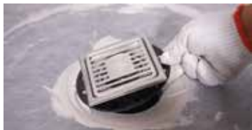
Install the drain adjustment ring
