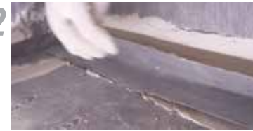
Cover the waterproofing strip
