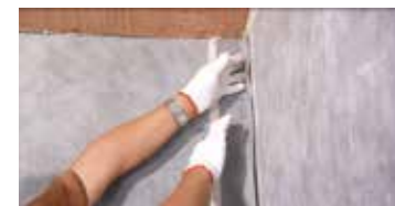
Cover the waterproofing strip on the corner
