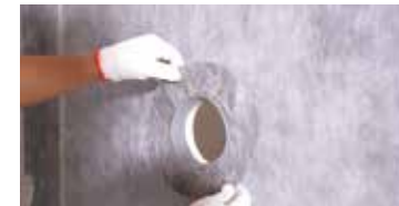
Cover the pipe seal
