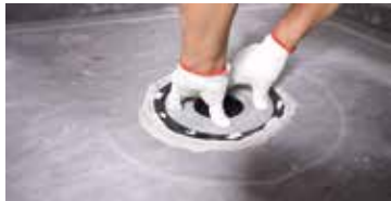
Rotate the flange to fix it firmly
