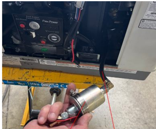
Incoming fuel line – pulling slack from outside the generator
