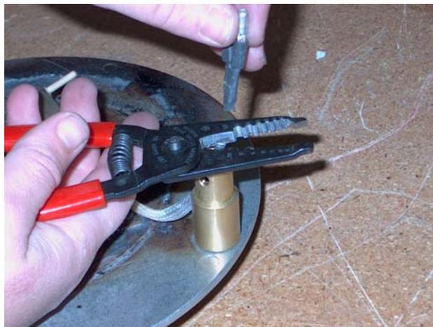
Cut old connectors from RTD, this will allow the RTD to be removed from the spacer.
