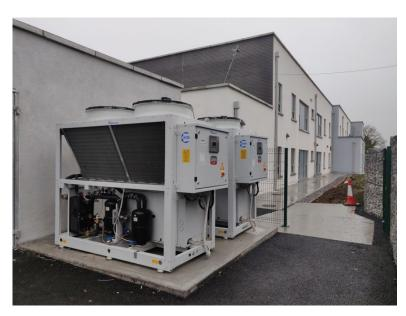
These supply a 1500L buffer tank and can meet the heat load of the building during most of the year.
