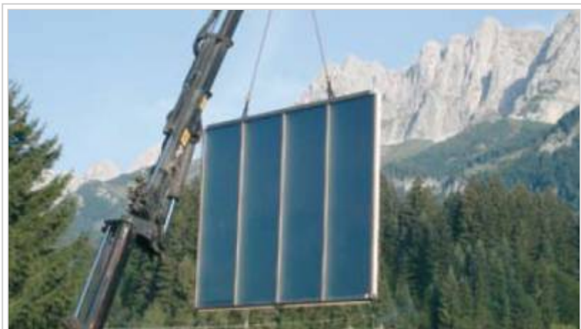
Large TiSun FA collector being lifted into position
