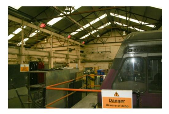
In such a vast complex of buildings, control of the operational hours and the temperature becomes of critical importance. Radiant sensitive blackbulb thermisters are used for picking up the temperature data which is relayed back to controllers within each individual building. This arrangements ensures that there is no wastage of natural gas and that the employees can start the working day in a comfortable environment.
