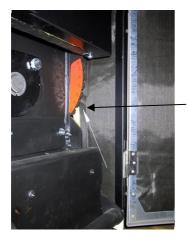
Setting the air adjuster on the front of the boiler on the right above the small ash box.
