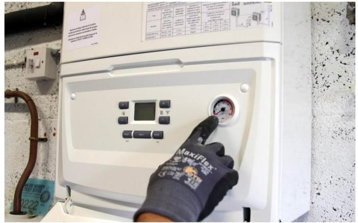
Replacing the existing boiler was straightforward as the pipework required little modification. Pipe locations and centres on the Magis Combo Plus are similar to those on all Immergas boilers.
