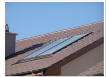
Flat Panels on a roof
