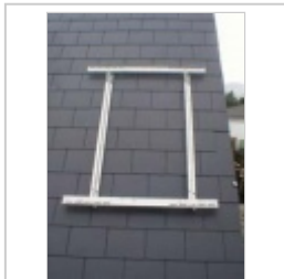
The completed frame
