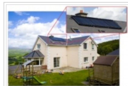
Solar Panels on a roof
