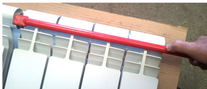
Figure 4 —Joining key
