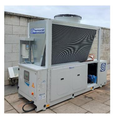
The Domino SEA 175Z is a commercial three-phase air/water chiller equipped with EC axial fans and hermetic scroll compressors.
