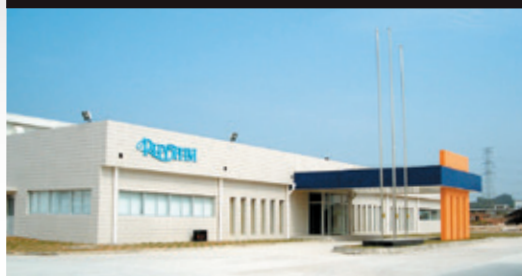
● THK RHYTHM GUANGZHOU CO., LTD. (China) Site: 23,000m 2 (247,570sq.ft.) / Floor space: 8,900m 2 (957,988sq.ft.)
