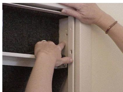
8. Pull back interior felt lining inside Quick Vault to locate installation holes, there are 2 on each side, on the hinge side the holes are toward the front, and are not threaded
