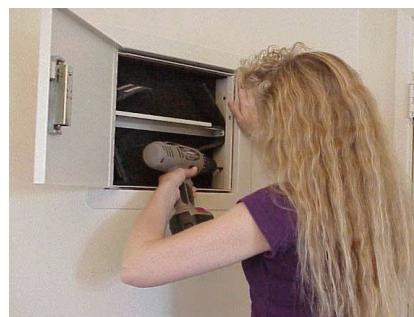
9. Pre-drill holes into studs for screws
