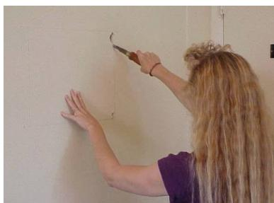
4. Cut dry wall in between wall studs
