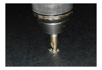
Remove the vault from the vehicle and drill a 1/2" hole where the 1/8" pilot hole was drilled.
