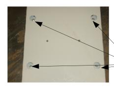
3. Anchor SIP plate to floor with the provided bolts.
