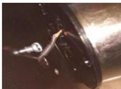
Ensure that the lock cable is positioned so that it lies in the channel on the back of the lock. This channel is provided to protect the lock cable from damage or crimping during installation.
