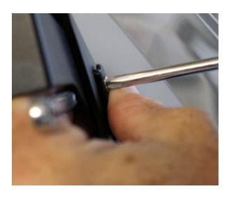
Use the 7 mm open wrench and the Phillips screwdriver to pre-tighten the arm plate to the bracket – just enough so you can swing the mount to attach it to the other side.
